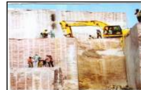
Doddamuduvadi Granite Quarry
