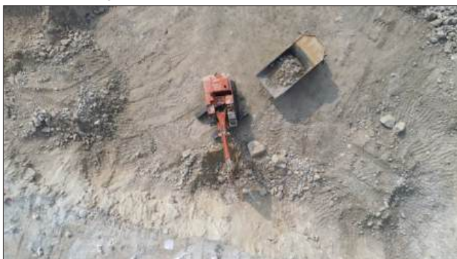
Fig 1. Load and Haul Operation
