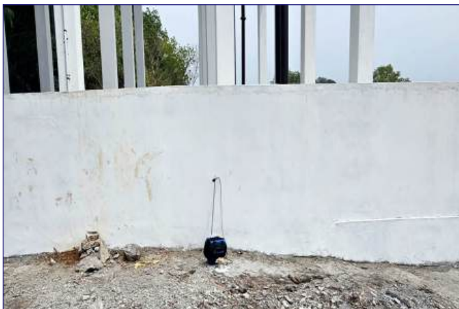
5. GROUND VIBRATION MONITORING NEAR THE WATER TANK
