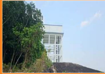
2. VIEW OF WATER TANK
