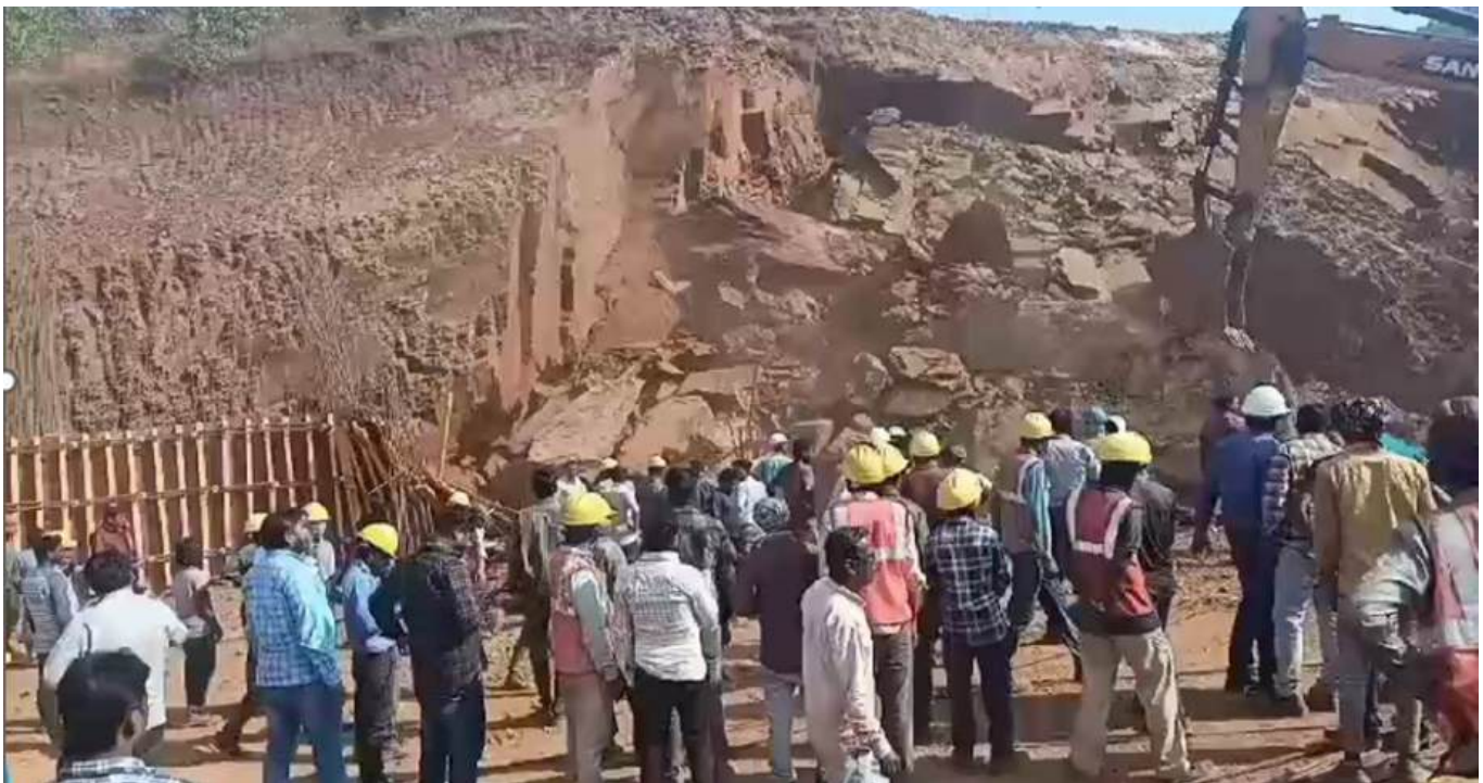
6. Recent instability at Kirandul Iron ore mine The undercutting of the wedge might have led to the sudden and catastrophic failure
