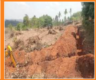
4. A VIEW OF TRENCH CREATED
