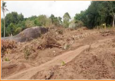
1. BROAD VIEW OF THE QUARRY
